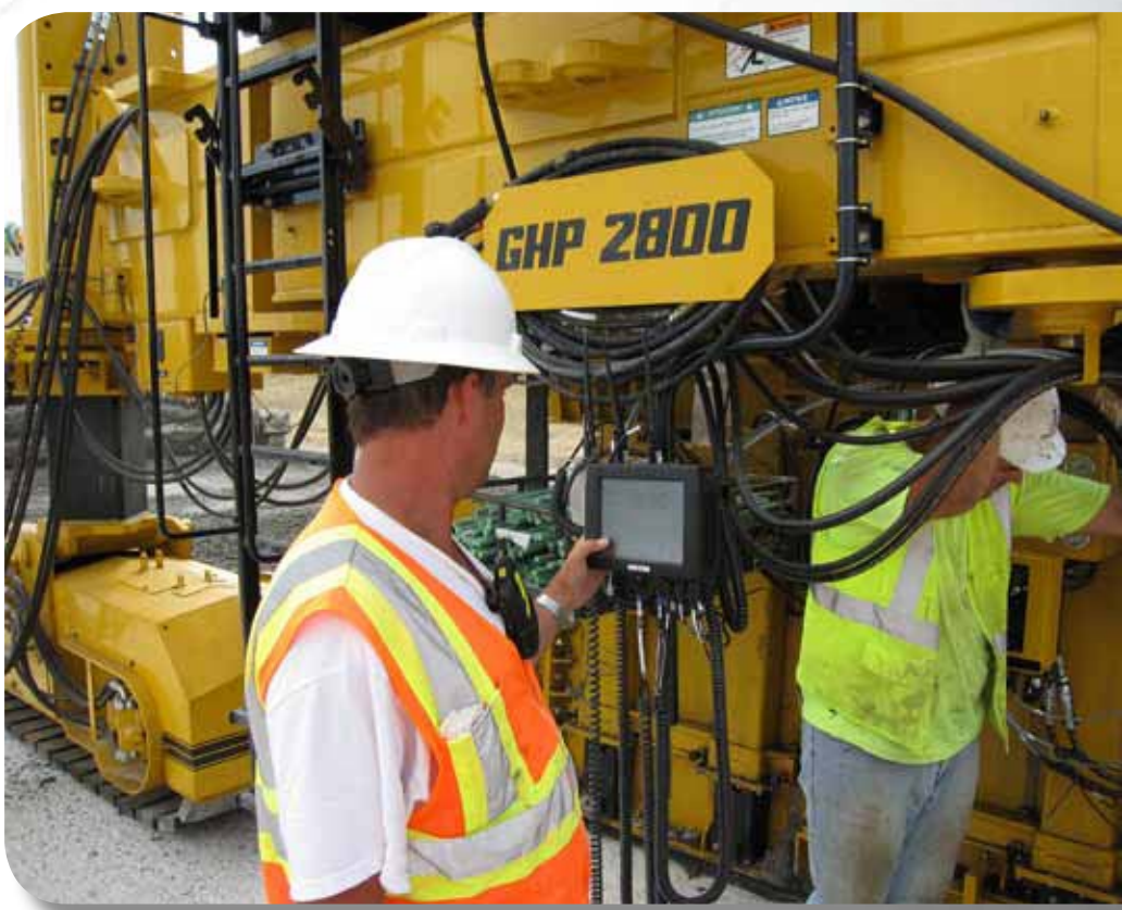
John VanMeter of Leica GeoSystems shows how the system is started on the GOMACO 2800 Paver.
